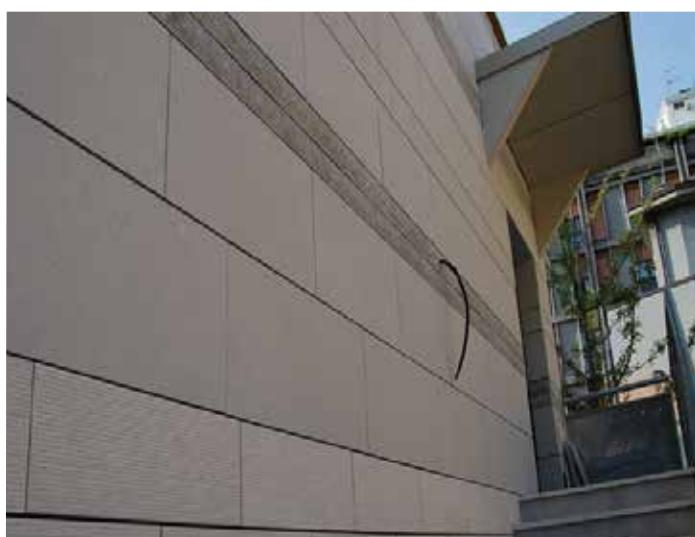
*The constructive technology of Vertech is based on slabs placed onto a metallic and aluminium structure constituted by a network of easily adjustable steel sections in order to obtain perfect complanarity and vertical facade.*
